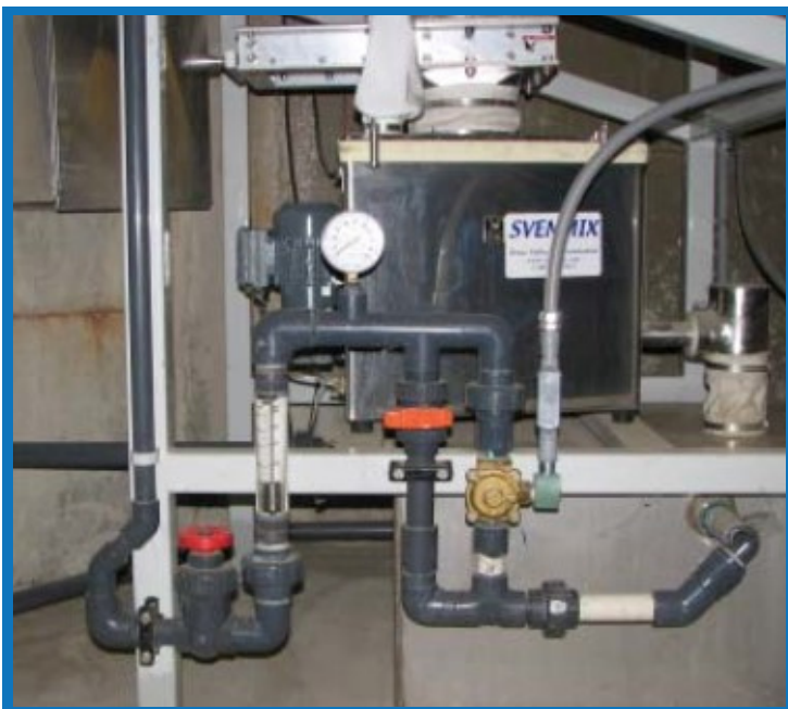
SVENMIX DTM Volumetric Feeder, Dissolving Tank and Mixing Water Controls
