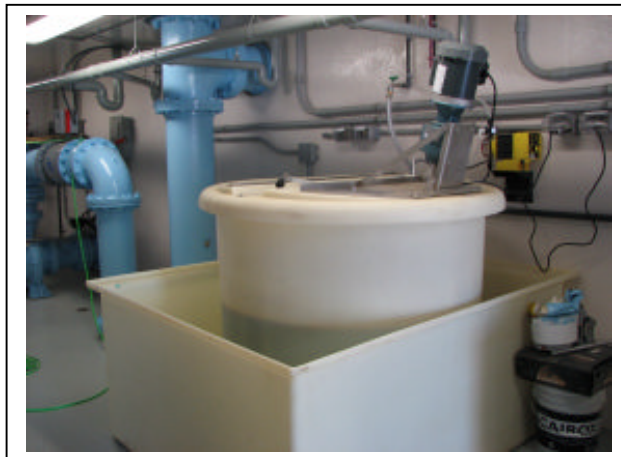
SVENMIX 300Gal. Graduated Cross-Linked Polyethylene TANK with SVENMIX LS MIXER and SECONDARY CONTAINMENT
