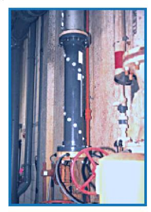
SVENMIX INJECTION RINGS can be an integral component of the SVENMIX STATIC MIXER or a stand-alone unit to provide an even distribution of chemical solution into the sludge stream.
